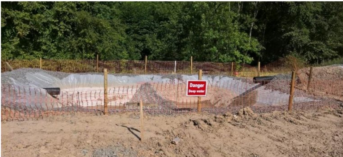
Figure 5-3 Example of settlement ponds
