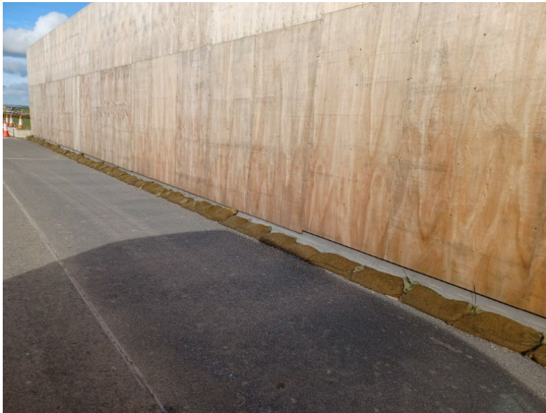
Figure 5-4 Anti-spillage elements installed along a bailey bridge
