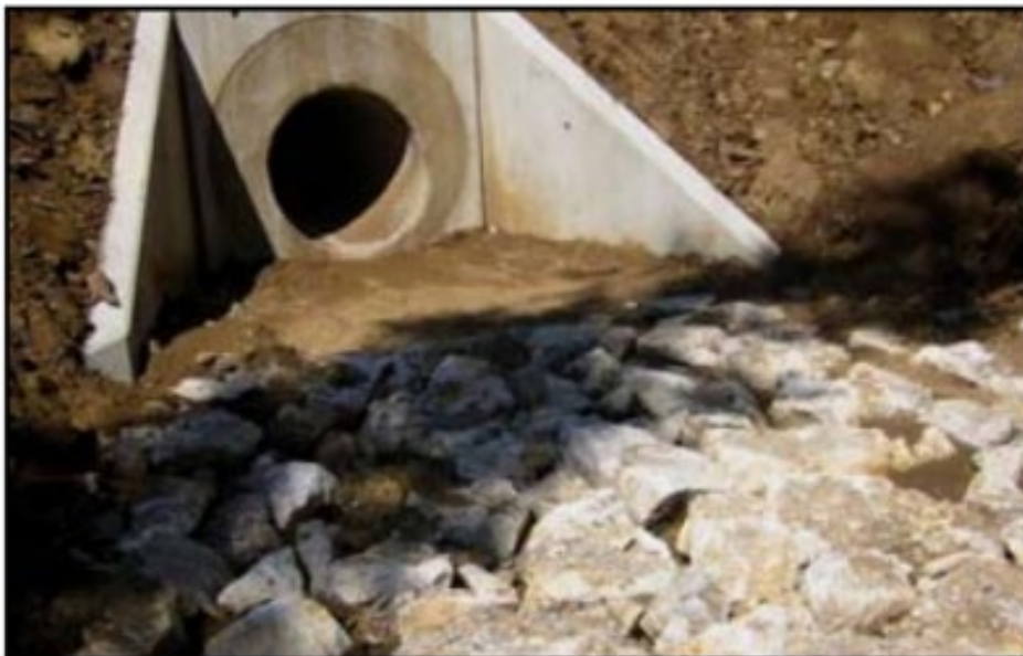
Figure 3-2 Rip rap protection of outlets
