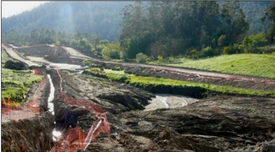
Figure 3-1 Temporary cut-off ditches
