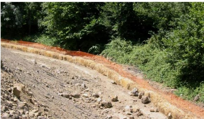
Figure 5-1 Example of a straw bales barrier for prevent spread of loose material.
